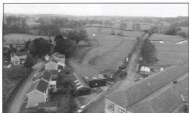
Left: Lowerhouse from the top of the Mill chimney.
